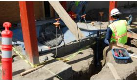
Electrician installing the conduit pipes in the elevator mechanical room foundations
