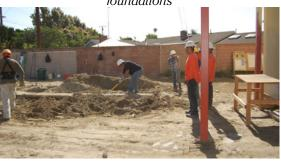
Using sledgehammers to break concrete footing
